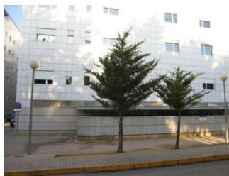
Hospital P. Socorro.
